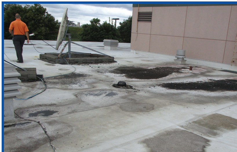
Above, the roof at Cataract School.
